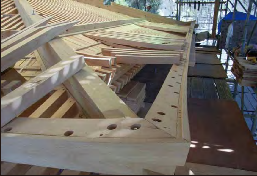
17 茅負、飛檐垂木取付
